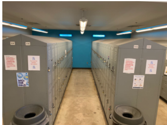
Figure 3 START Coalition shelter in Oklahoma showing UR UVGI fixture commissioning and deployments (Source: Equity Air member Bill Palmer of AeroMed)
