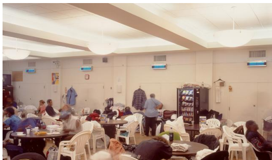
Figure 2 TUSS New York City Shelter Showing UR UVGI fixtures on the wall in a 24 h/7days drop-in center where many persons stayed. (Source: TUSS)
